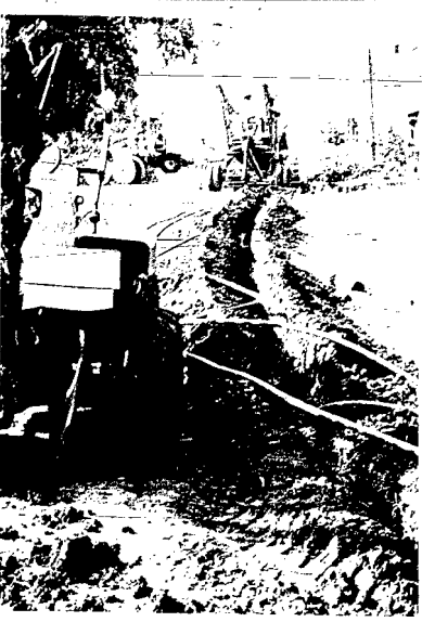
Lots of wire is going into the ground at Dixon as workmen improve the telephone system there.
